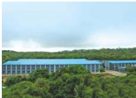
DG Set Manufacturing Unit-Kalsar, Gujarat
