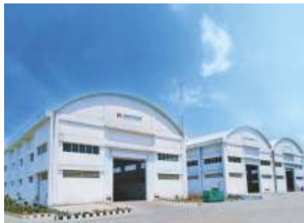
DG Set Manufacturing Unit 1-Kathua, J&K
